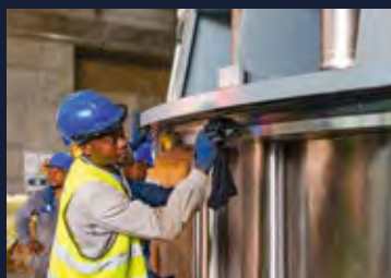
📍 Nachtigal Hydropower, Cameroon
