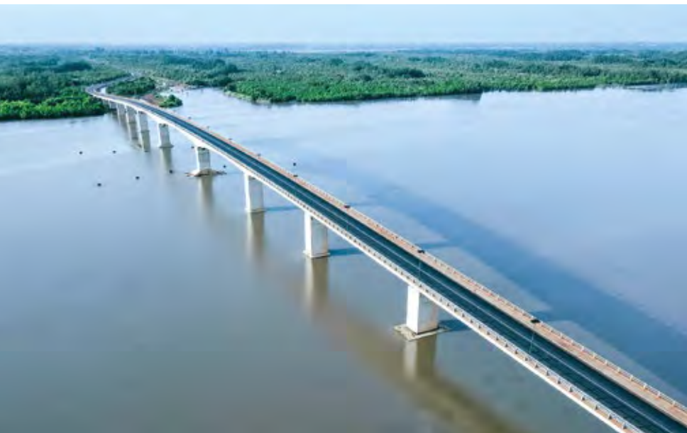
Senegambia Bridge, The Gambia
