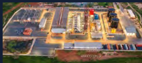
Malicounda Power Plant, Senegal
