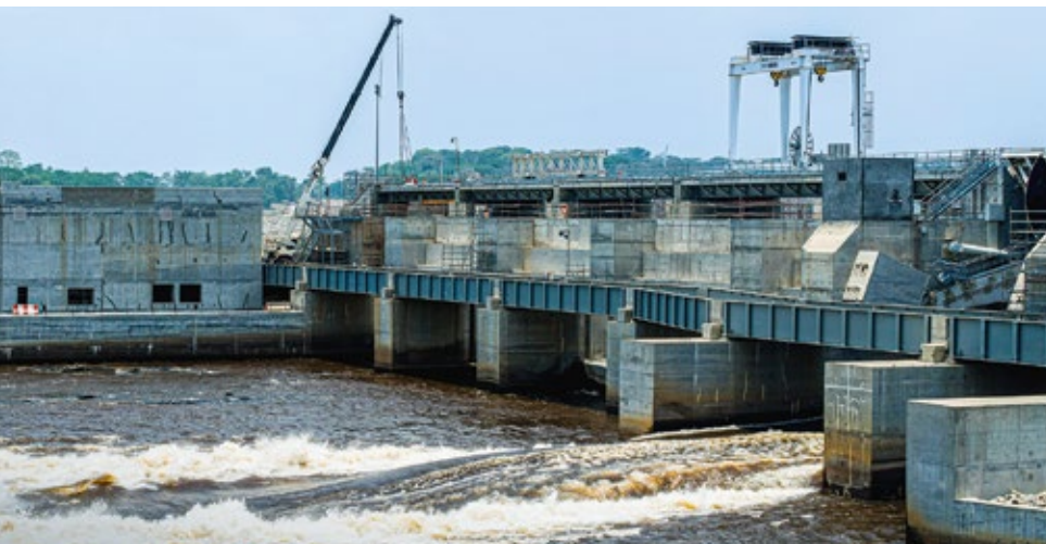
🌿 Nachtigal Hydropower, Cameroon
