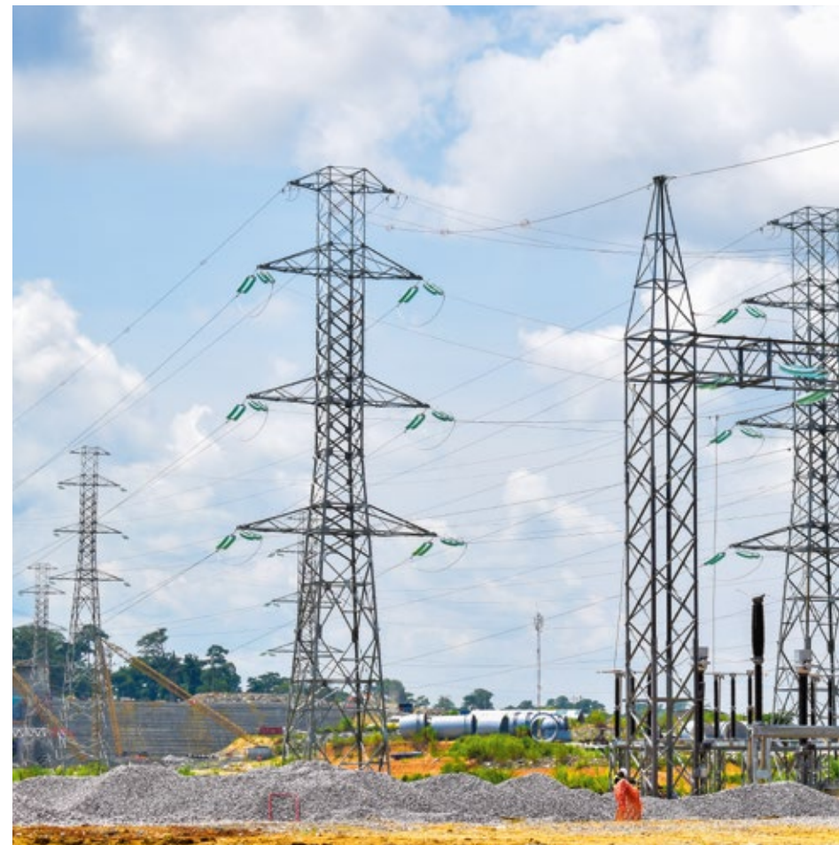
📍 Kenya Transmission PPP Project, East Africa
