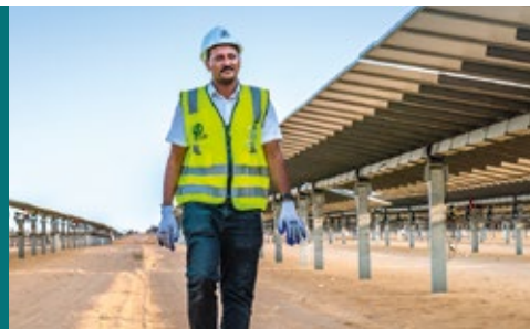
Benban Solar Park, Egypt
