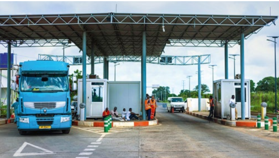
📍 Senegambia Bridge, The Gambia
